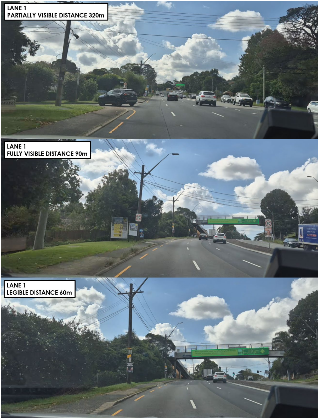
Figure 2.5: Warringah Road Eastbound Approach Sign Exposure – Lane 1
